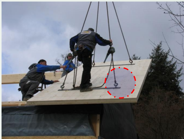
mounting parts for roof elements
