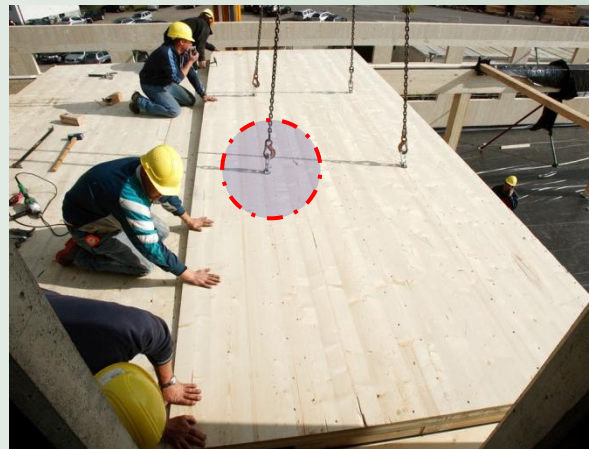
mounting parts for ceiling elements
